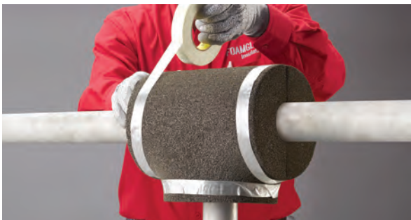
Use of factory pre-fabricated fittings
