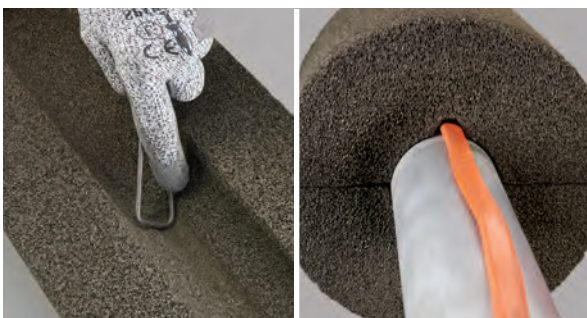
Application over trace heating
