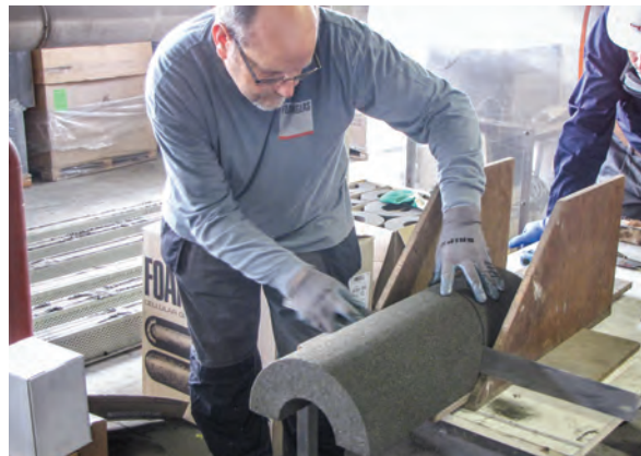
TESSENDERLO, BELGIUM, TRAINING CENTER DEMONSTRATION
