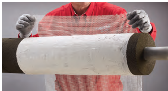
Application of scrim and mastic
